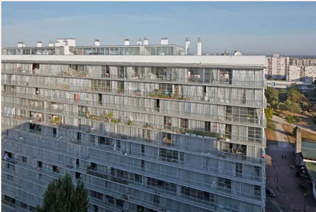
The repurposed Grand Parc 1960s estate, in Bordeaux, was upgraded rather than demolished © Philippe Ruault
