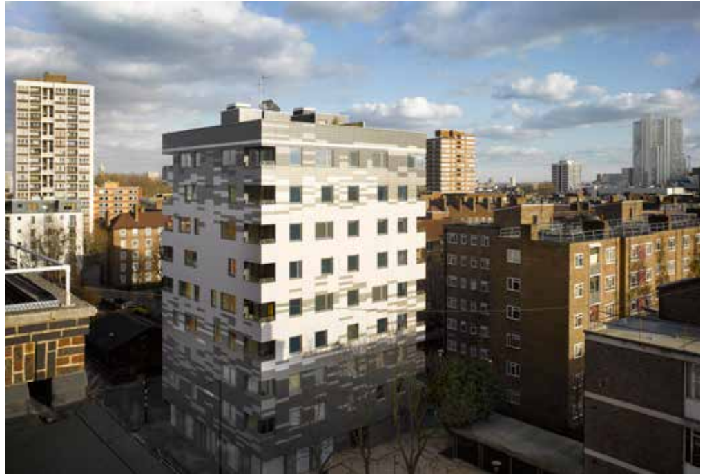
Lightweight wood pulp cladding covers the timber structure with pixelated panels Photo: Will Pryce
