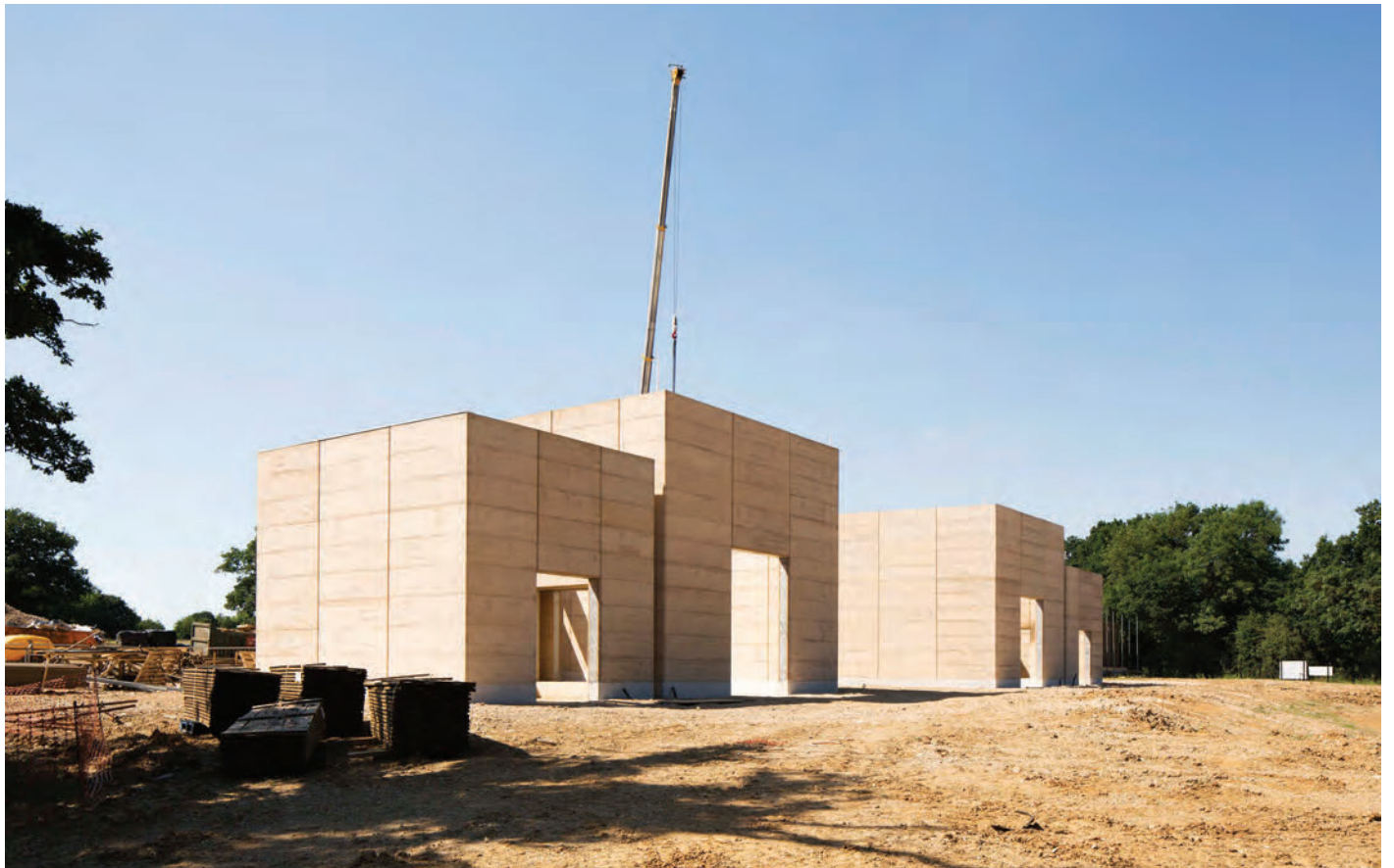
Above Steel goalpost structures were cast into the rammed earth walls to provide openings for the prayer halls large Cor-ten steel doors Top left Visualisation of the completed project Above right and below Construction of the 7m-high walls was completed in July
