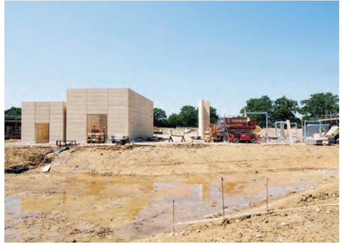
Above Steel goalpost structures were cast into the rammed earth walls to provide openings for the prayer halls large Cor-ten steel doors Top left Visualisation of the completed project Above right and below Construction of the 7m-high walls was completed in July
